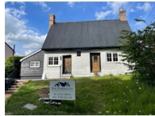
Period Restoration & Listed Buildings
